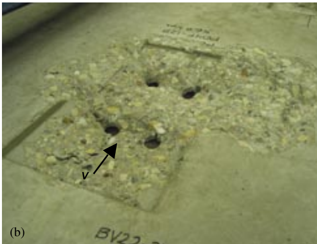
Fig. 11. Failure conditions of Test PO4F-12B with y = 6 in. (152 mm): (a) Deformation of studs after test; (b) Perspective view of the concrete breakout on the slab.
