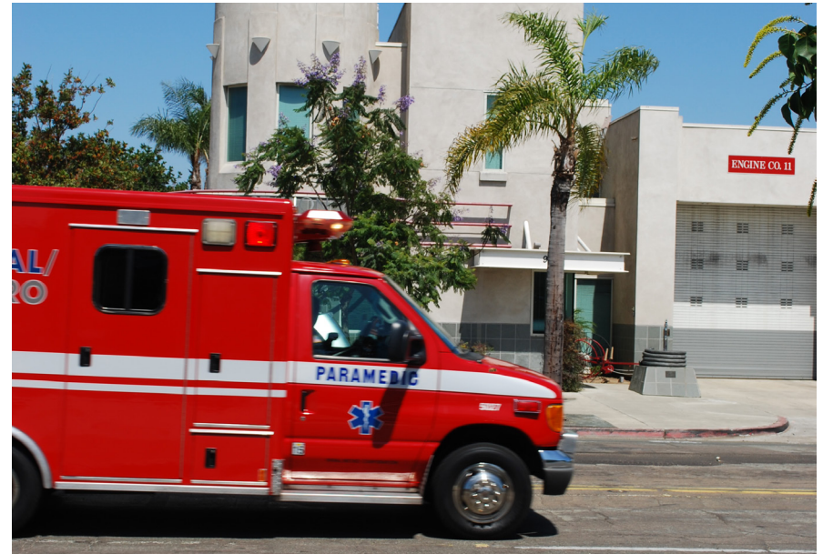
Fire Station 11 provides fire and medical emergency services to the community from its site at 25th Street and Broadway.
