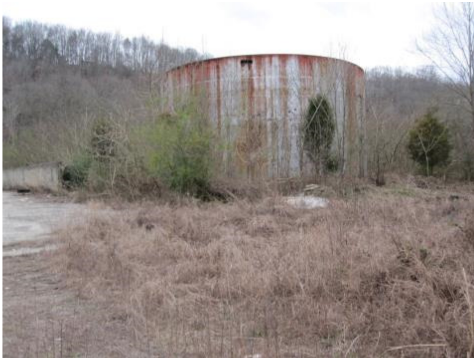
Photo 3 – Closer view of 630,000-gallon AST at the site. The landowner removed this tank in September 2014. Concrete retaining wall and drive at the left center of photo is being undermined by the Emory River. (Photo credit: Brad Parman, 03/11/13).
