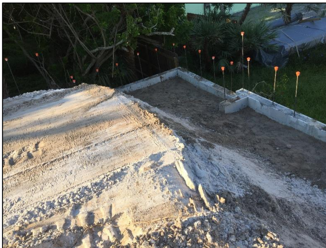
View from Top of Fill Dirt Pile
