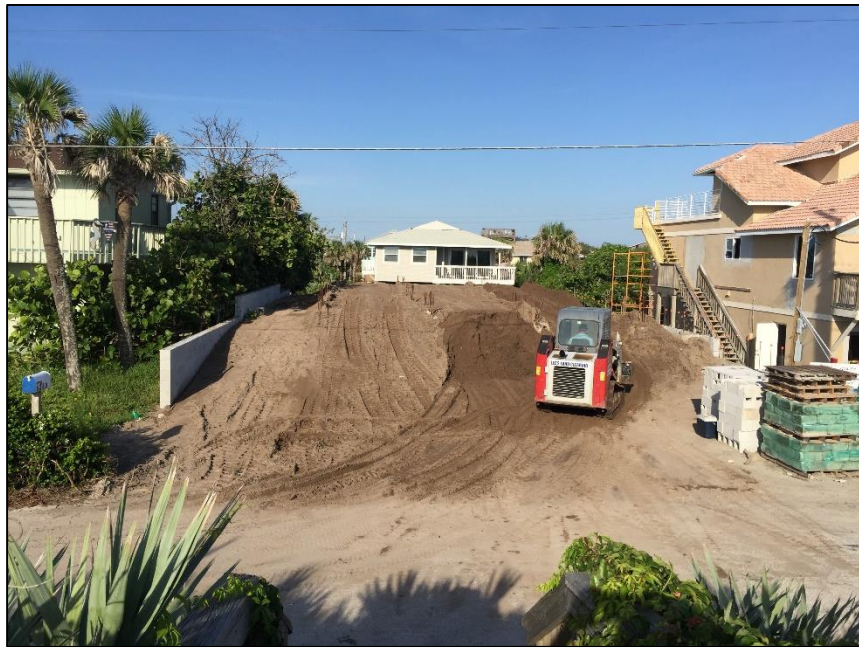
South Wall (Phase 1 Complete)
