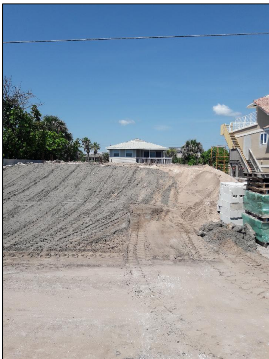
View from South Atlantic Avenue (Phase 1 Complete)
