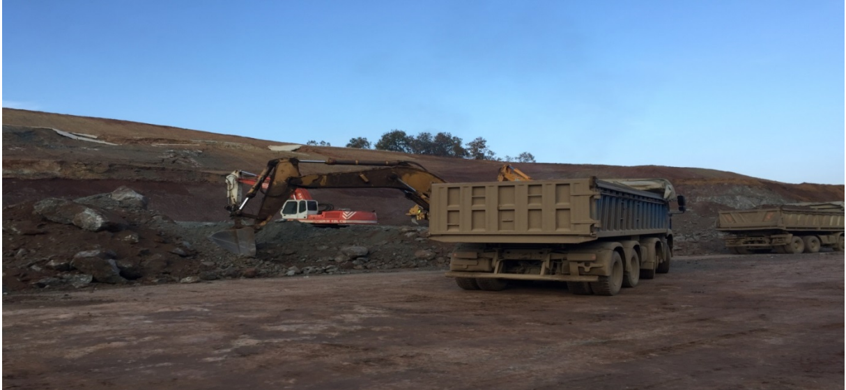
Figure 7 - Construction works at the E-65 Central Motorway in Greece
