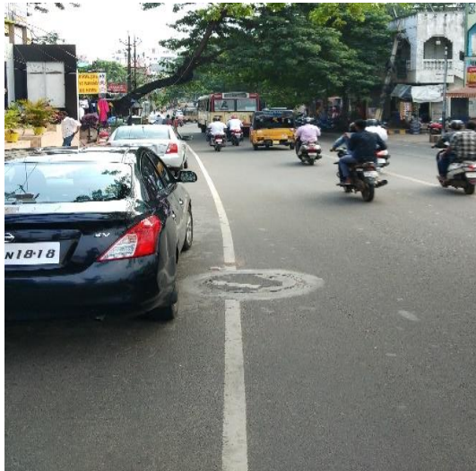
Fig. 20. Road stretch from Jagadamba-Jail road junction
