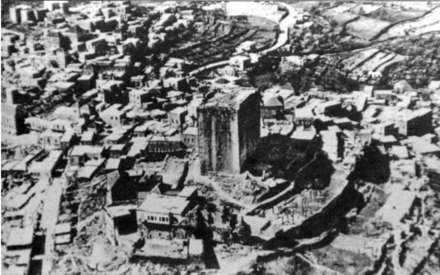
The tower of Castel Blanc (Burj Safitha) dominated the surrounding Syrian town. The 27m-high tower is a typical donjon and was rebuilt in the late-12th or early-13th century when it was occupied by the Templars. It is also one of the best-preserved Crusader fortifications in the Middle East. The ground floor served as a church, and continues to do so to this day. (Institut Francais d'Archeologie, Beirut)
