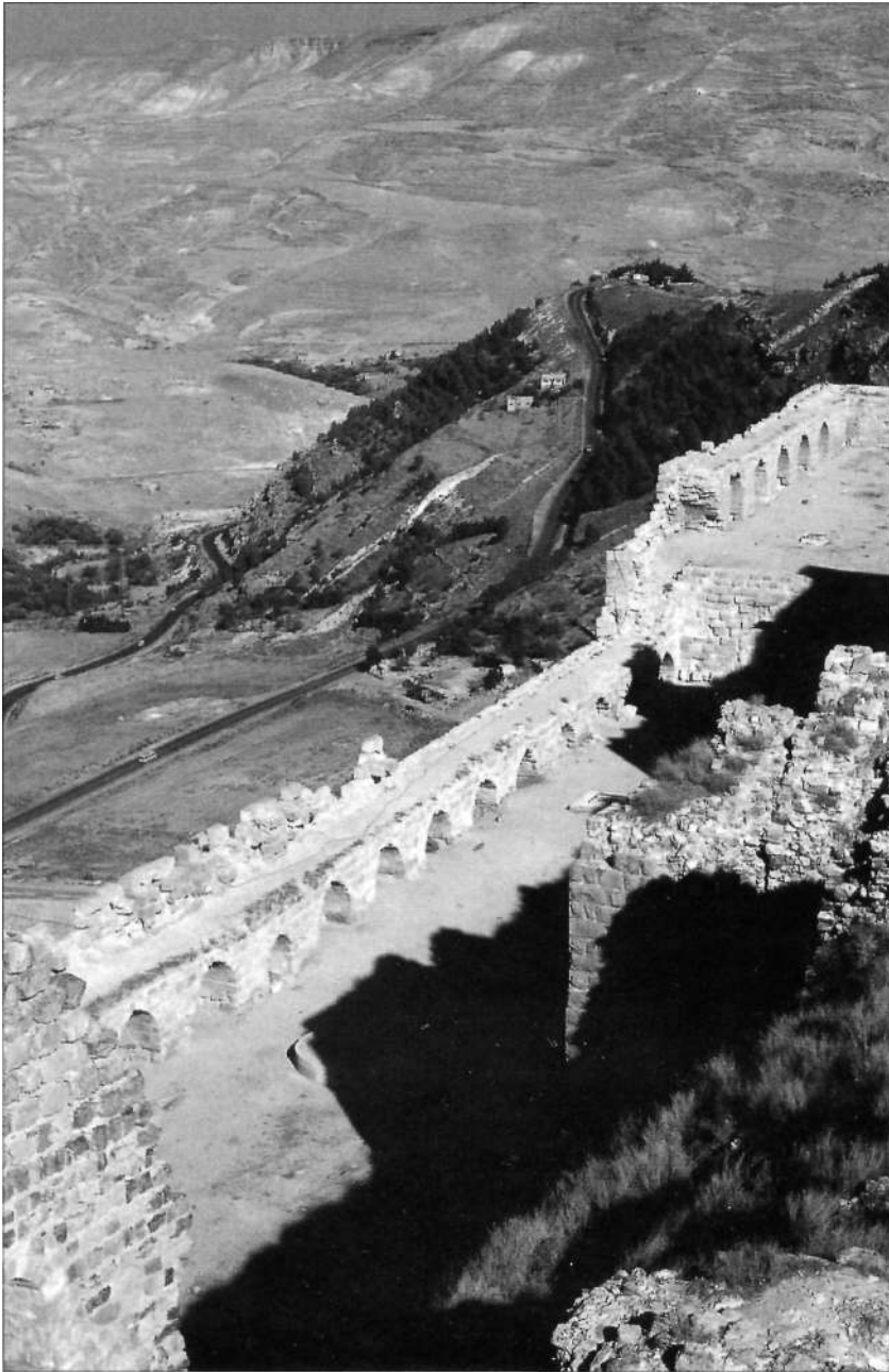
At least two stages in the construction of Karak castle are seen here. In the foreground are the remains of the walls and towers built during the second Crusader phase around 1168. Beyond and below it is a massive barbican dating from the Mamluk era in the late-13th and 14th centuries.
