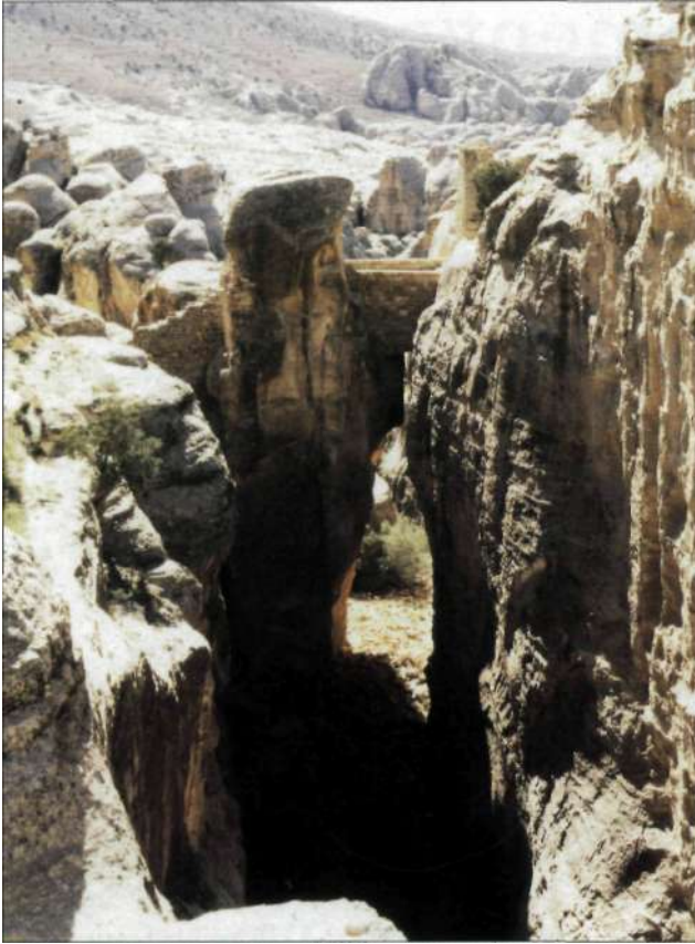
At al-Wu'aira the builders of the Crusader castle widened and straightened an existing rocky gorge rather than excavating a fosse from the rock. The anvil-shaped outcrop in the centre of the picture was then pierced with a tunnel to make an outer gate. The stone steps and bridge that now link this rock outcrop to the castle on the right and the other side of the gorge on the left are modern. In the 12th century there would have been a drawbridge and a removable wooden bridge.
