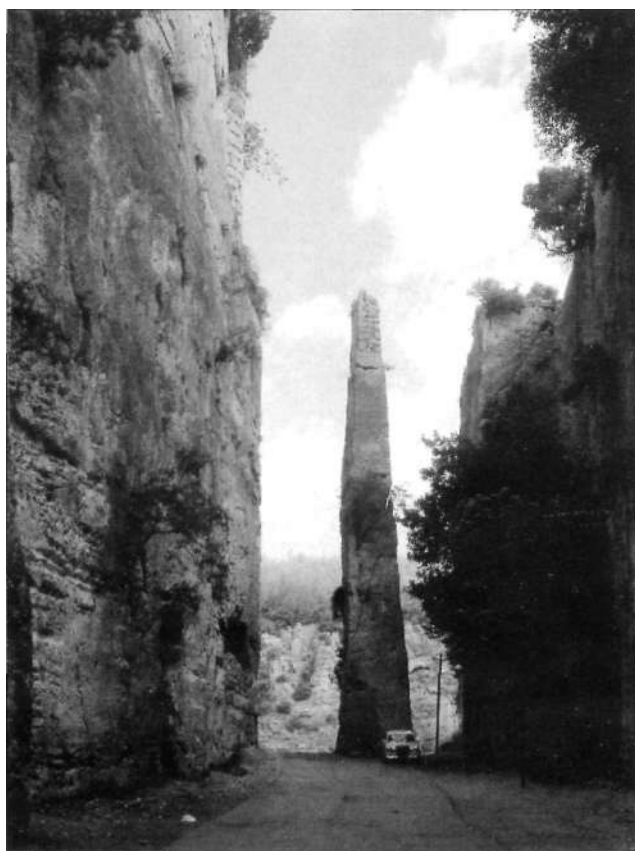
ABOVE LEFT The needle of rock that was left in place when the Crusaders, or more likely the slaves and prisoners of war forced to work for them, excavated the remarkable fosse at Saone. The fosse separated the castle, on the left, from the rest of the hill on the right, while the pillar itself originally supported a bridge.
