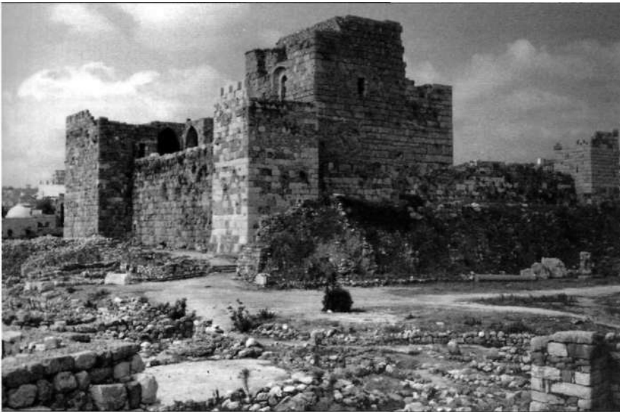
The citadel of the castle of Gibelet (Jubayl) consists of a four-sided enclosure with corner towers, with a separate keep in the centre. It was built by the Crusaders early in the 12th century, and although changes were made in the 13th century the overall character of Gibelet's fortifications remains simple. (D. Pringle)
