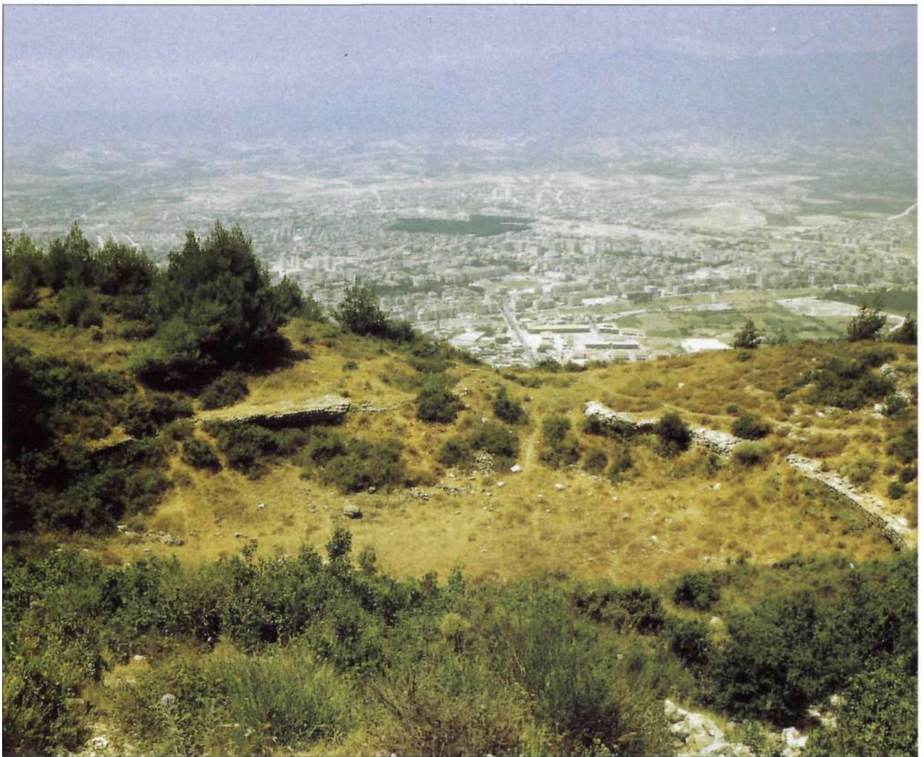
The oval-shaped open water cistern near the Crusader Citadel at the summit of the fortifications of Antioch. The retaining wall would originally have gone all the way around.
