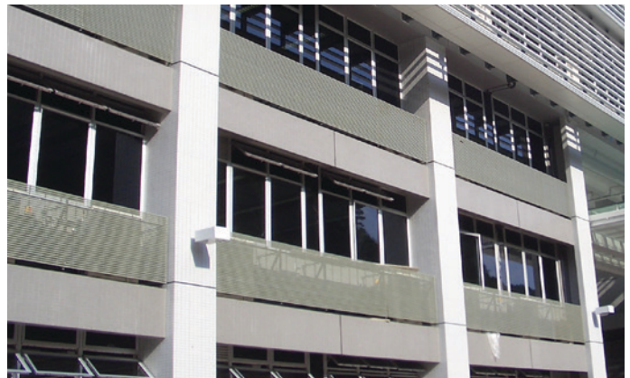
Strongwell I-6000 grating was installed at this School of Business and Information Systems in Hong Kong as air-conditioning platforms when placed horizontally and as louver when placed vertically (as shown here).
