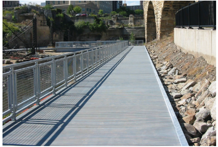
Mill Ruins Park in downtown Minneapolis, Minnesota utilized T-1800 1" for new pedestrian walkways in the beautiful historical district.
