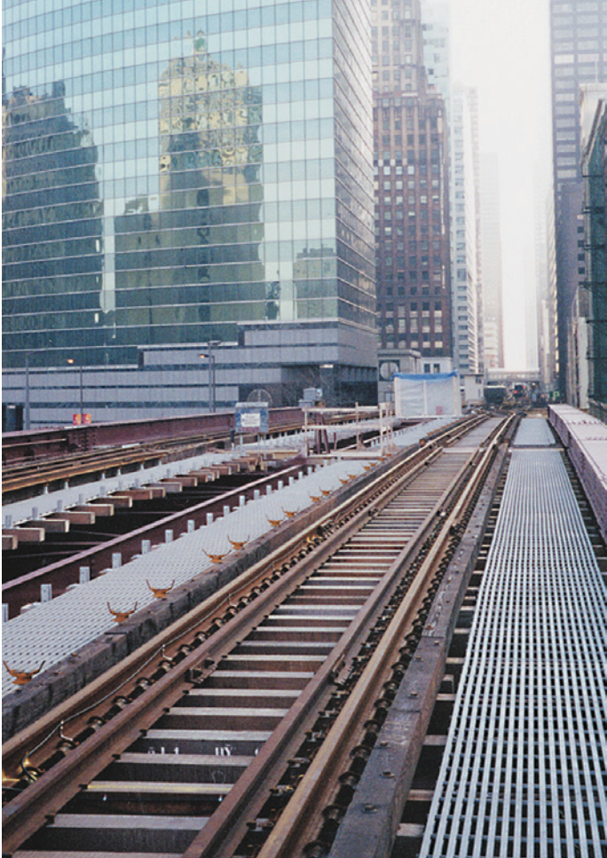
Chicago Transit maintenance walkways alongside elevated train tracks constitute one of the largest fiberglass grating installations in history. This project used T-5000 2" with a custom polyester resin.
