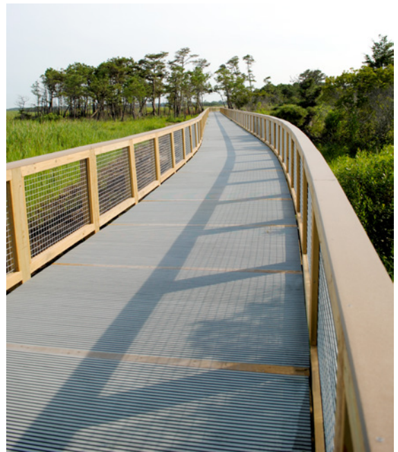
Almost 5,000 panels of I-4000 1" were used to create a nearly half-mile walking and biking path at Cape Henlopen State Park near Lowes, Delaware.
