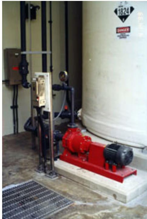
Figure 4. Close-up of one of the two sealless thermoplastic magnetically-driven centrifugal pumps automatically delivering the required volume of 25% NaOH on demand.
