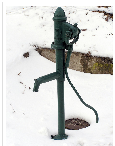
Hand-operated, reciprocating, positive displacement, water pump in Košice-Ťahanovce, Slovakia (walking beam pump).
