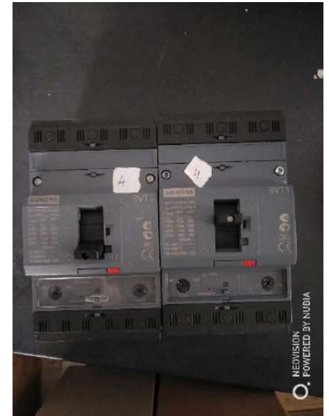
Molded case circuit breaker 3VL
