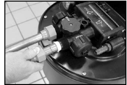
Figure 4: Connect Water Lines
