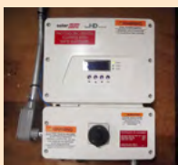
Figure 56A. Stand-alone inverters convert DC power from batteries into AC power.
