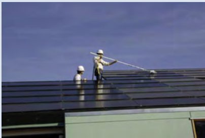
Figure 108. Cleaning soiled PV arrays is a common maintenance need.
