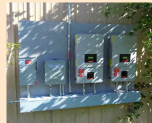
Figure 56B. String inverters are small inverters in the 1 to 12 kW size range, intended for residential and small commercial applications.
