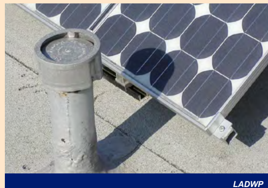
Figure 17. Shading of PV arrays can be caused by any obstructions interfering with the solar window.
