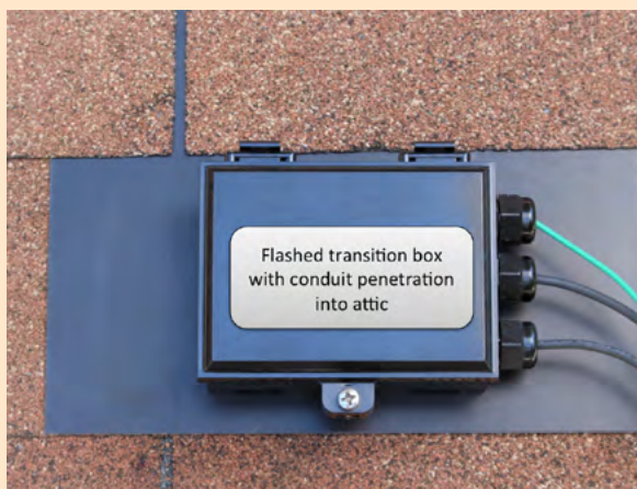
Figure 97. Flashed transition box
