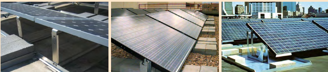
Figure 22. Self-ballasted PV arrays are a type of rack mount that relies on the weight of a the PV modules, support structure and additional ballast material to secure the array.
