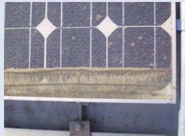
Figure 108. Cleaning soiled PV arrays is a common maintenance need.
