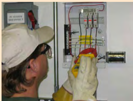
Figure 101. Operating parameters in PV systems are measured to verify expected performance.
