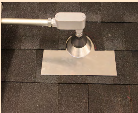
Figure 96. Flashed conduit penetration
