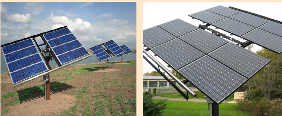
Figure 24. Sun-tracking arrays can be mounted on poles and increase the amount of solar energy received.
