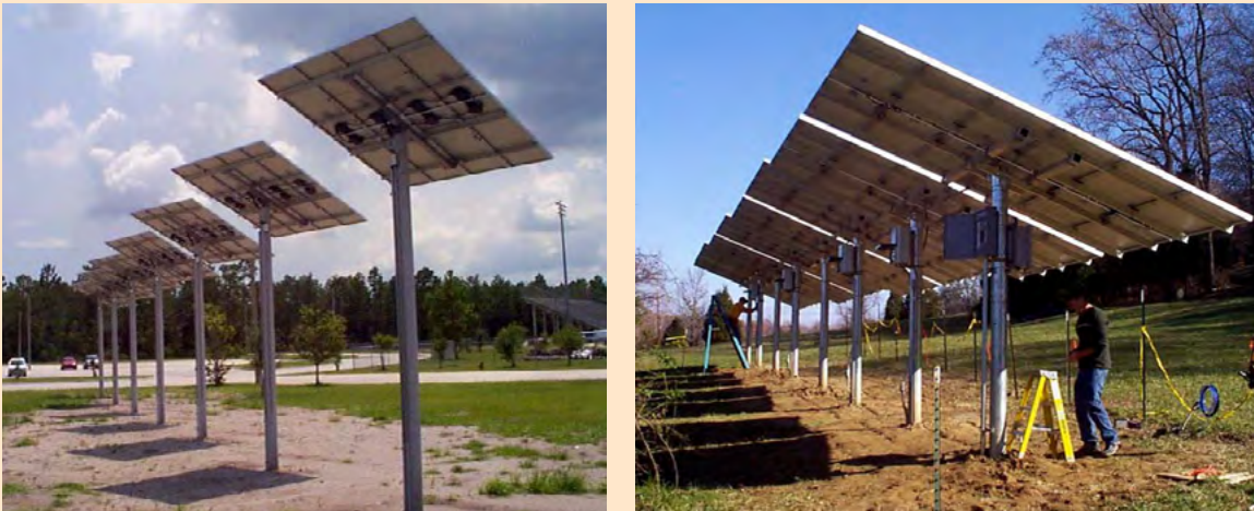
Figure 23. Pole-mounted arrays use either fixed, adjustable, or sun-tracking arrays installed on a rigid metal pipe.
