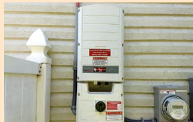
Figure 56B. String inverters are small inverters in the 1 to 12 kW size range, intended for residential and small commercial applications.
