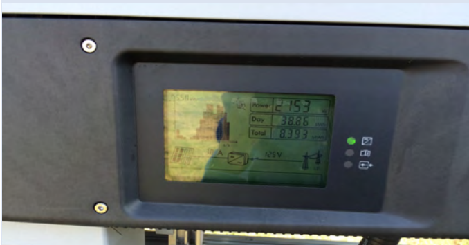
Figure 105. Inverter Display
