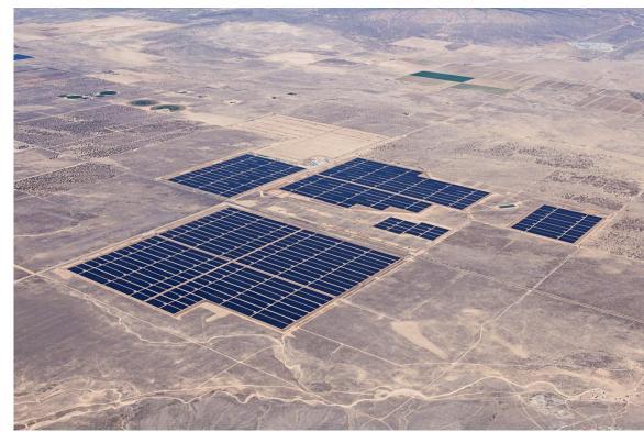
Antelope Valley, CA, USA 579MW 1,720,000 PV panels Over 600 inverters
