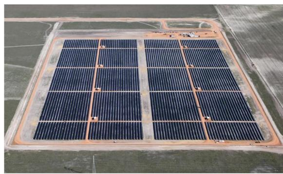
Greenough River, WA, AU 10MWp 150,000 PV panels 16 x 720kW central inverters
