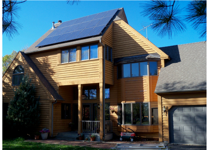
Residential PV solar installation in Minnesota
