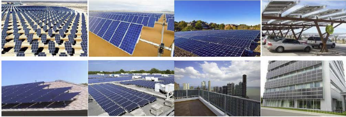
Figure 42: Examples of some of the deployment designs being considered for bifacial PV systems.
