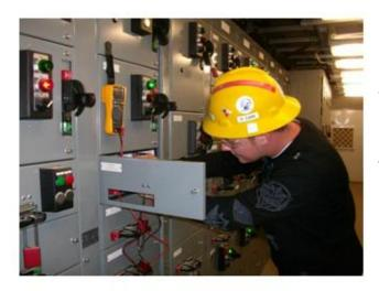
Voltage, continuity checks and destructive testing are verified for proper start up.
