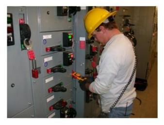
Amp checks to ensure and verify proper amp draw of equipment.
