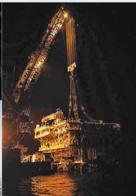
Platform 19A of Iran's South Pars gas field (in the Persian Gulf) was installed over Phase 19 of the gas field on Saturday night. Phase 19 is set to produce 56 million cubic meters per day of sweet gas, 75,000 barrels per day of gas condensate, 400 tons a day of sulfur, 1.05 million tons a year of liquefied petroleum gas and one million tons a year of ethane.
