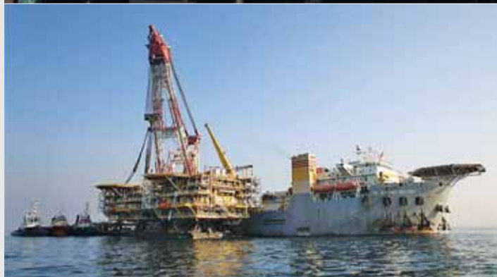
Platform 19A of Iran's South Pars gas field (in the Persian Gulf) was installed over Phase 19 of the gas field on Saturday night. Phase 19 is set to produce 56 million cubic meters per day of sweet gas, 75,000 barrels per day of gas condensate, 400 tons a day of sulfur, 1.05 million tons a year of liquefied petroleum gas and one million tons a year of ethane.
