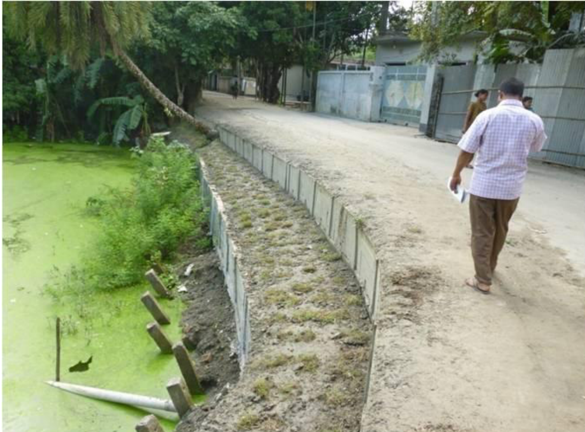
Figure 3: Slope protection and road improvement in Manikganj Pourashava
