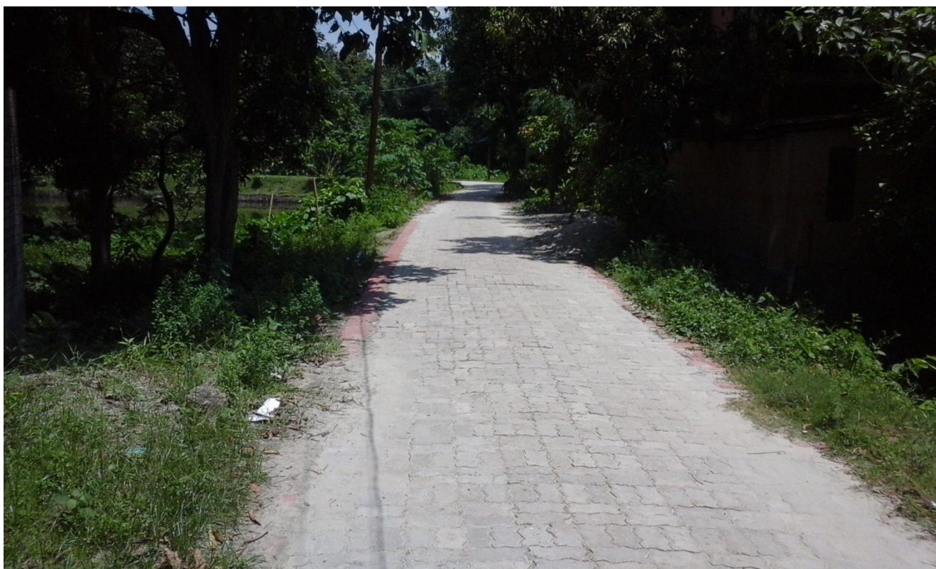
Figure 6: Uni-block (Concrete block) road in Sonargaon Pourashava
