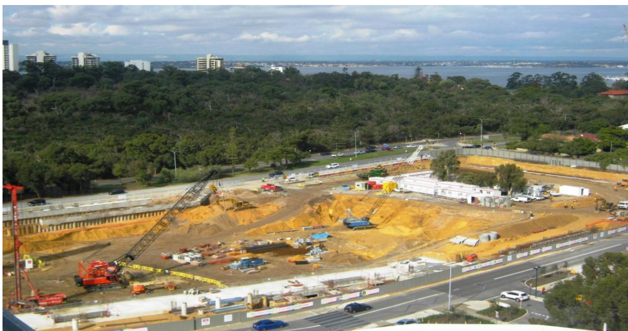
New Children's Hospital construction site – May 2012
