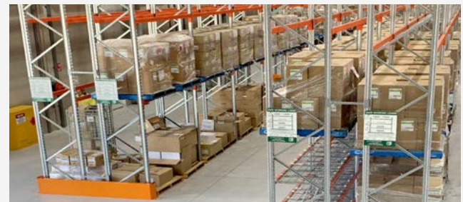
New regional warehouse in Rockhampton commissioned
