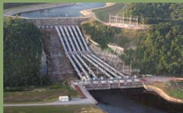
Salina Pumped Storage Project and W.R. Holway Reservoir Salina, OK - 1968 Units 1, 2 and 3 - 130 MW
