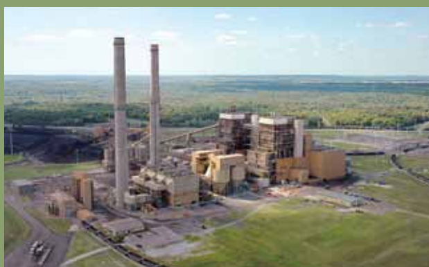
Coal Fired Complex - Chouteau, OK Unit 1 - 490 MW, 1982 Unit 2 (GRDA's 62%) - 322 MW, 1985
