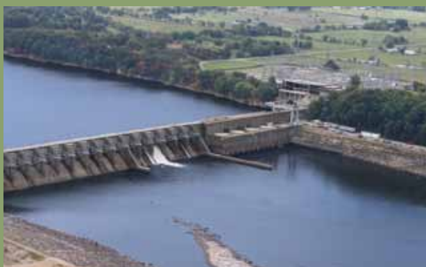
Robert S. Kerr Dam and Energy Control Center Locust Grove, OK - 1964 Units 1, 2, 3 and 4 - 108 MW
