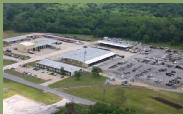
Transmission and Distribution Headquarters Pryor, OK
