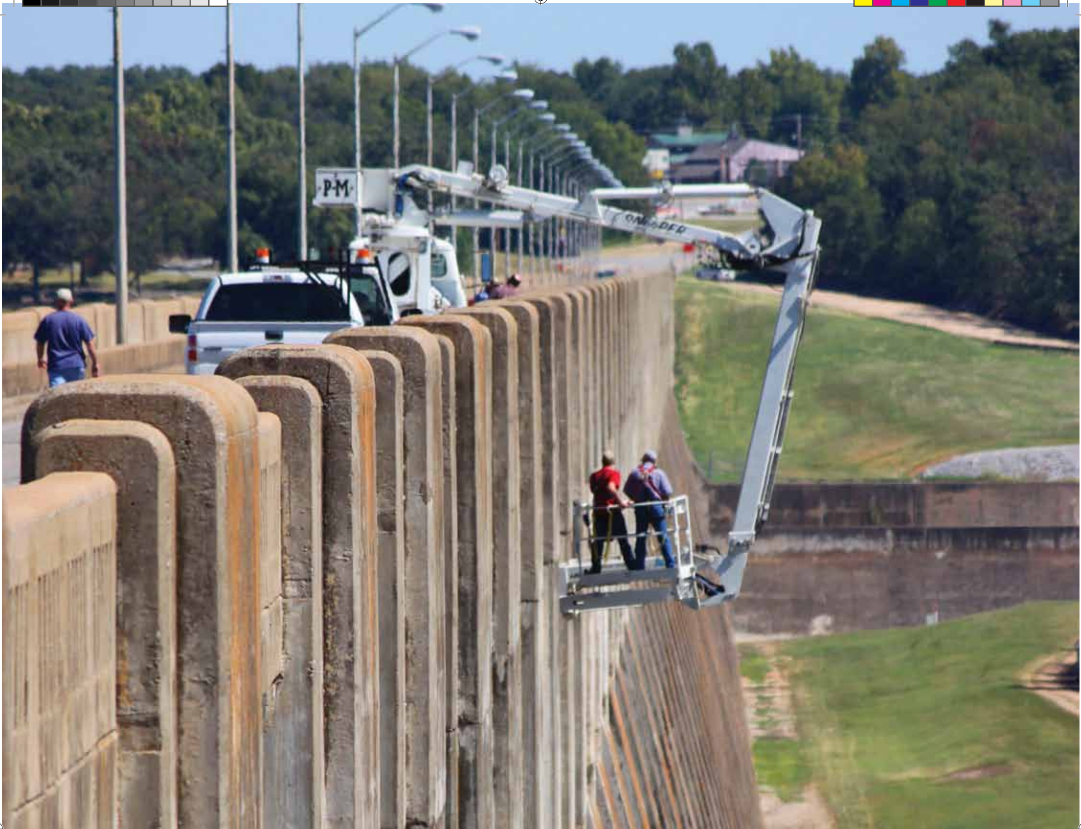
PENSACOLA DAM INSPECTION
