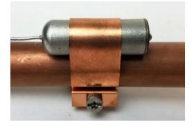
Thermostatic expansion valve sensing bulb placement and mounting
