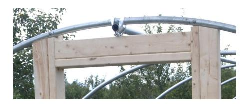
Hold a 2X4 horizontally across the inside of the top of the doorway. Place one edge of it against the left inner door frame board and behind the right door frame boards. Using the right door frame board as a guide, make a mark on the 2X4 on the inside edge of the frame. Cut 2 pieces of 2X4 to this length.
