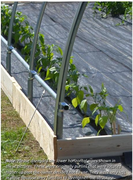
baseboards there. Predrill with a ¼-inch drill bit through the ground posts and thru-bolt with ¼"-20 X 3" carriage bolts and nuts. A thicker material was chosen for these baseboards because they will support the door frames and act as door jambs, which will likely get stepped on and take frequent abuse.
