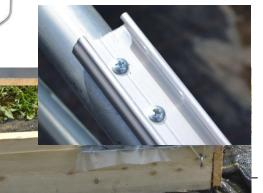
hipboard. Center it vertically and clamp it in place. Using #8 X ½-inch Phillips-head self-drilling tech screws, secure it in place. Phillips head screws are used to prevent damage to the plastic. Install screws every foot or so. Butt a second piece up to the end of the first and secure in place. Repeat down both sides of the tunnel. Use a hack saw or reciprocating saw to cut the final pieces to length prior to attaching.
