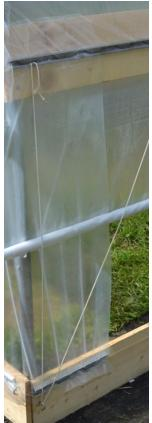
On the side of the tunnel, pull the bottom end of the plastic tight and poly latch wire a 2-foot section into the end of the hipboard and the small section of poly latch wire channel on the side baseboard below it.
