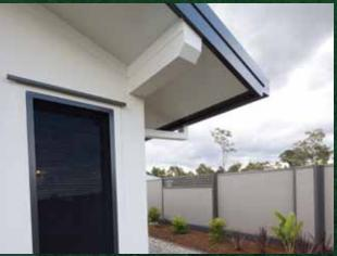
InsulWall's specially coated BlueScope Steel shell provides a flat surface, ready for rendering externally and painting or tiling internally, showcasing InsulLiving's potential for a perfectly flush finish.
