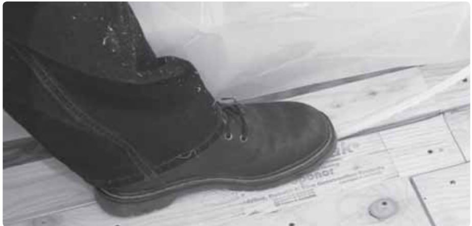
Figure 22: Use hard-soled boots or shoes to walk the tubing into the panel groove.
