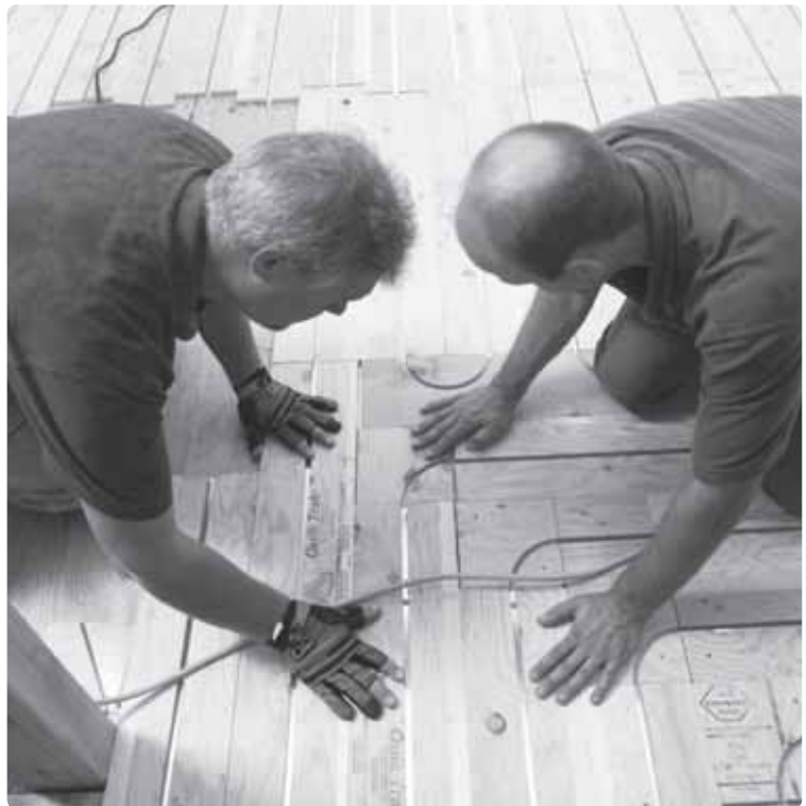
Figure 4: Installing Quik Trak Panels
