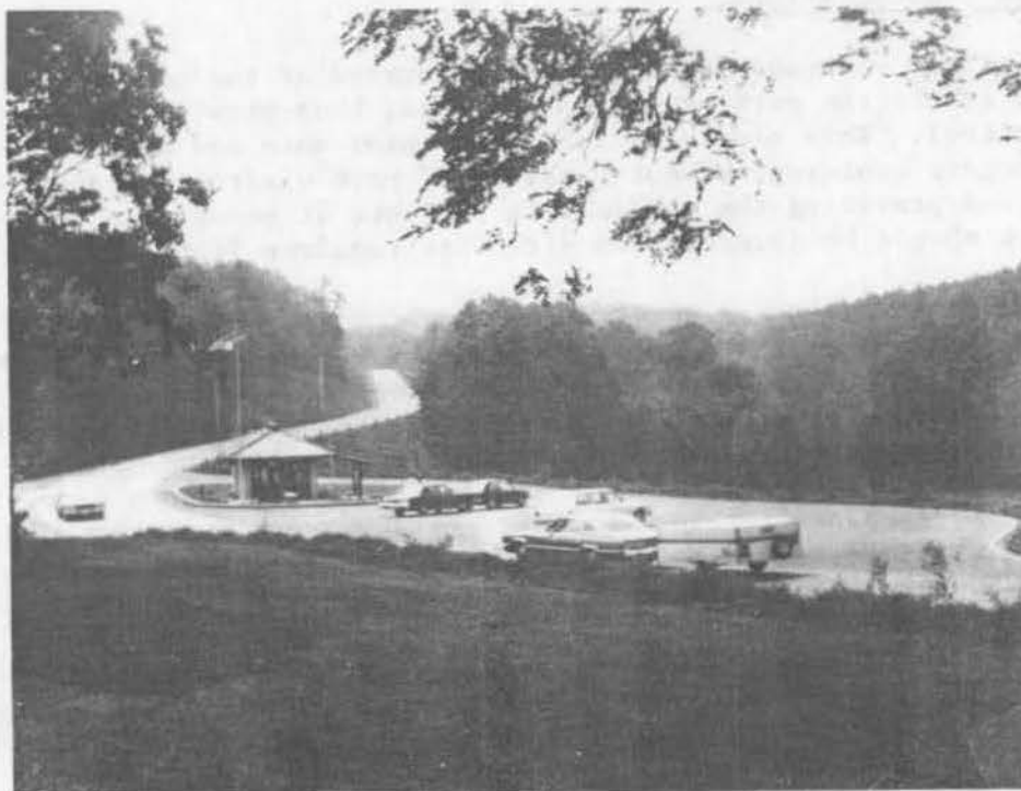
Figure 8-1 Typical entrance station to a recreation site
