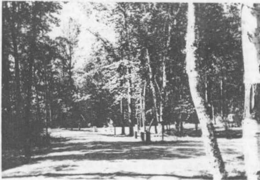
Figure 2-9 Grading for Recreation Roads in Activity Areas
