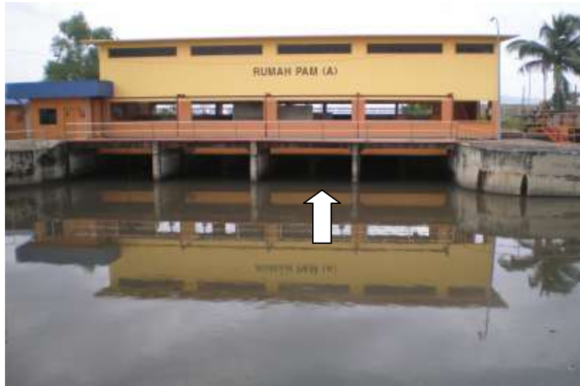
Fig 1. Inlet of a Pump A house.
