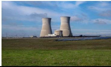
Rancho Seco Nuclear Generating Station SMUD
