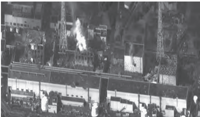
Figure 1-5 Fukushima Power Plant after the meltdown March 24, 2011—The composition of the gas escape cloud is a key determinant for the safe evacuation distance from the nuclear plant.
