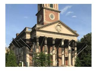
Figure 4. Safety Net Around Building (Photo by C. Lee)
