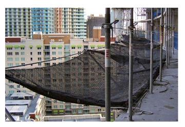
Figure 5. Safety Net Construction Site (InCord, 2019)
