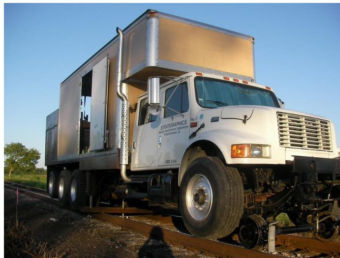
Figure 15: Stratigraphics CPT truck outfitted with High Railers performing penetration testing on an existing trackbed in Wisconsin (Stratigraphics)
