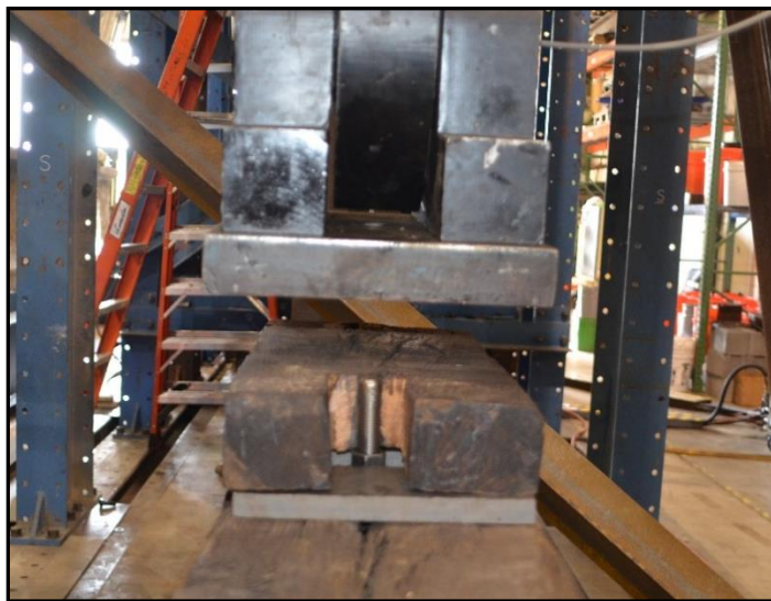
Figure 3-16: Wooden block used to allow steel plate to lay above hook bolt
