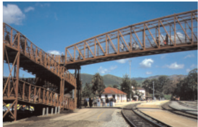
Trail-rail overcrossing. San Luis Obispo, CA
