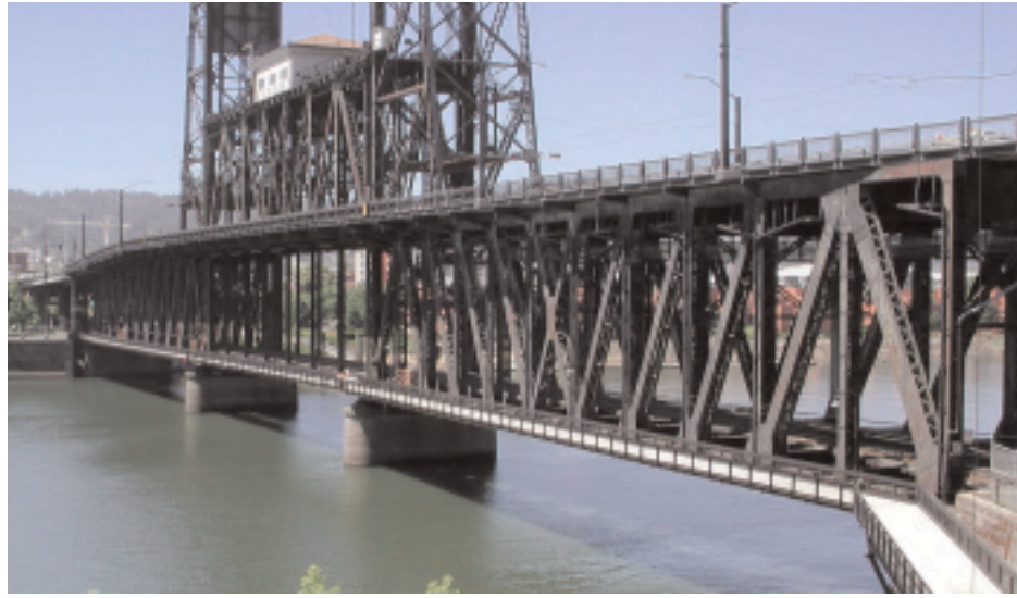
Steel Bridge Riverwalk. Portland, OR
