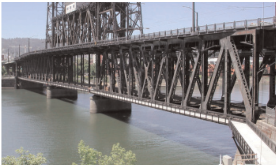
Steel Bridge Riverwalk. Portland, OR
