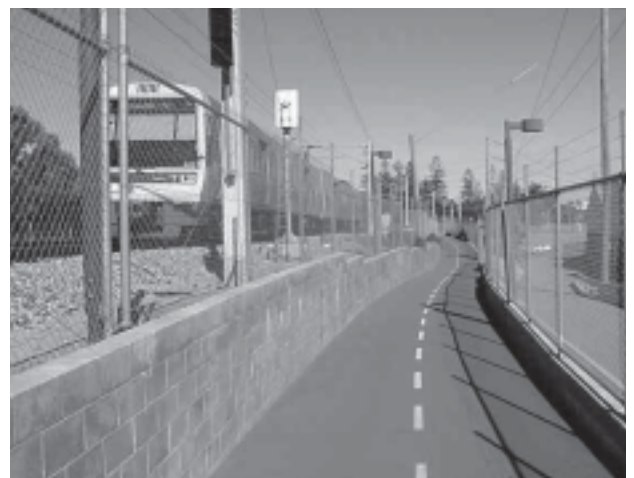
Setback (4.5m/15ft) and fencing along the Showgrounds Pathway RWT. Perth, Australia
