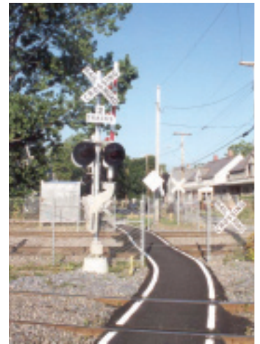
Dual track grade crossing. Burlington, VT
