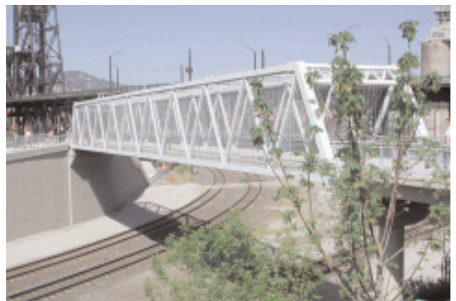
Overcrossing of Union Pacific tracks, Eastbank Esplanade. Portland, OR
