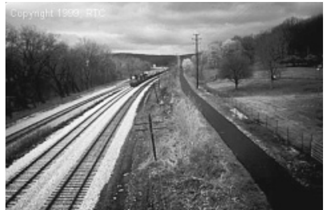
Setback of 7.6 m (25 ft) or greater often is needed for higher speed train corridors. Stavich Trail, OH and PA
