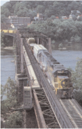
Harpers Ferry Bridge. Harpers Ferry, VA
