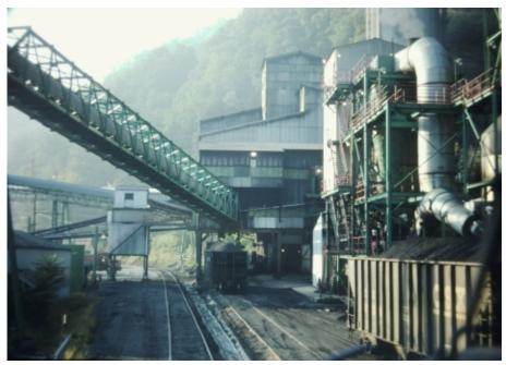
Prenter Mine - on the right are coal cars that have just been loaded. Under the tipple are two cars being loaded. Soon the management coal rider will roll them down to the other coal cars. When the loaded track is full they'll start using the empty track. When we first arrived and pushed empties up to the three track yard, we shoved them through the tipple on the track in front of our engine.
