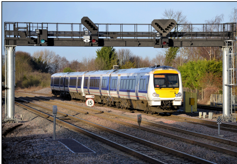
Figure 1: Train of Chiltern Railways approaching Princes Risborough station, showing various signals providing route control indications. Note also the fixed speed limit sign for movements over the crossover. Photo by Roger Marks.
