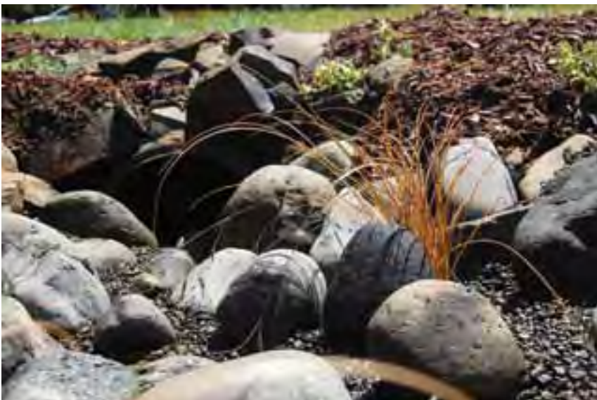
Figure 25: Rock, gravel, and sedges protect the inflow point in a rain garden. (Photo: Chris LaBelle, OSU)
