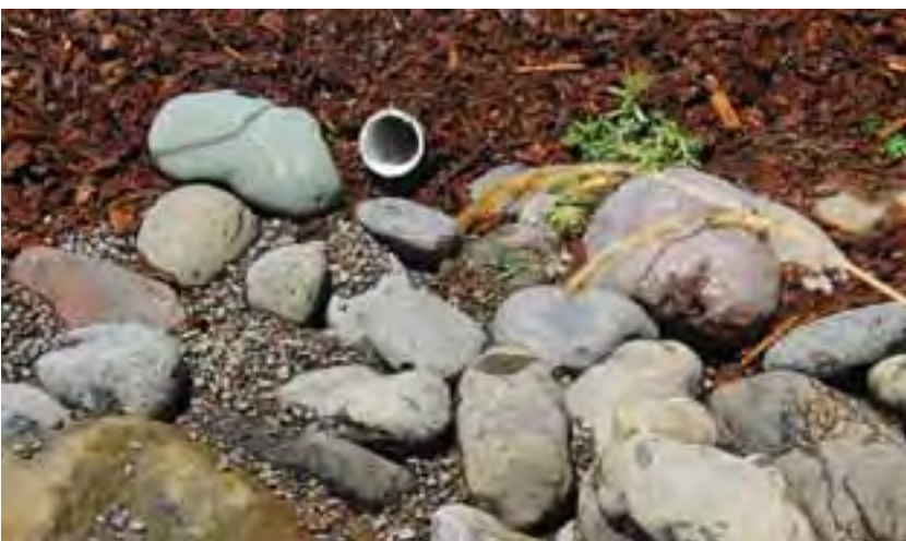
Figure 16: PVC pipe outflow from a coastal Oregon rain garden. The rocks, mulch, and gravel help protect the area from erosion. (Photo: Robert Emanuel, OSU)
