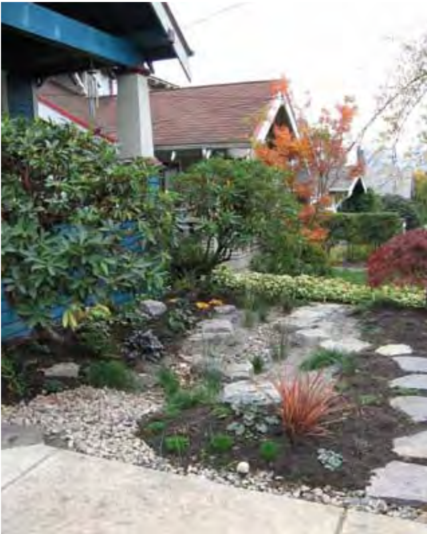
Figure 28: A rain garden that is mulched with gravel rather than bark. (Photo: Portland BES)
