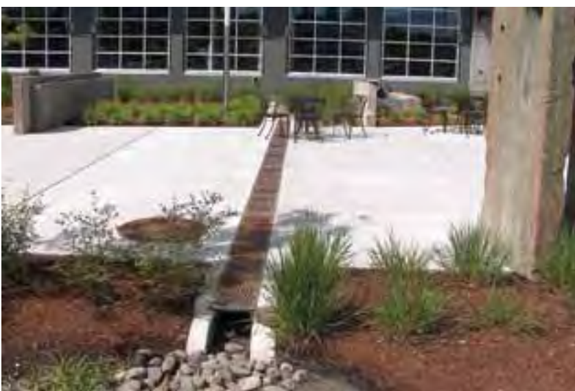
Figure 12: Trench drain through a sidewalk at a building in Portland. (Photo: Derek Godwin, OSU)
