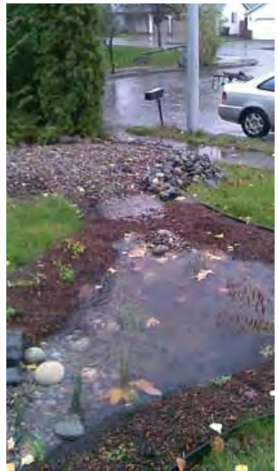
Figure 17: A rain garden in Gresham, Oregon, fills with rain. Note the use of rocks at the outflow point near top. (Photo: City of Gresham)
