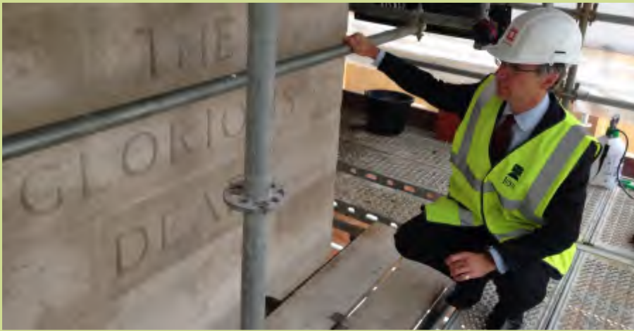
The English Heritage offered Dr Murrison the opportunity to visit the work being undertaken to restore the Cenotaph in preparation for the Centenary.
