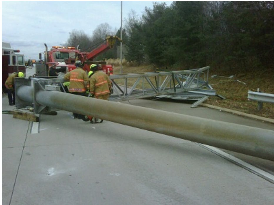
FIGURE 1 Sign structure collapse due to fatigue-induced anchor rod failure, Fairfax, VA (2012) (7).
