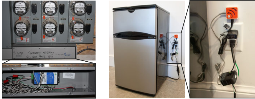
Figure 7. FRESH installed to support research in non-intrusive load monitoring (NILM): acquiring data from eGauge metering units in university housing via an API (Left), and metering a mini-fridge at the plug level (Right).
