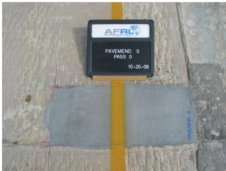
Figure 6. Typical Corner Spall Repair
