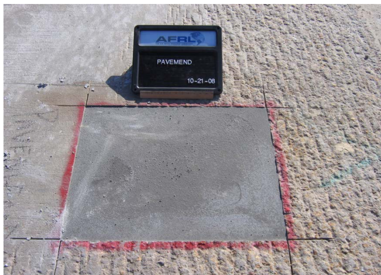
Figure 8. Typical Interior Spall Repair (Not Trafficked)
