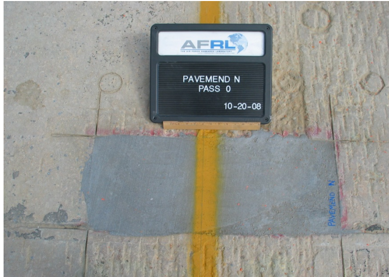
Figure 7. Typical Edge Spall Repair
