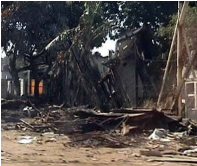
Figure 2 Wreckage of home reduced to rubble by Operation Murambatsvina ("Clean Up") June 8, 2005. Kubatana.net
