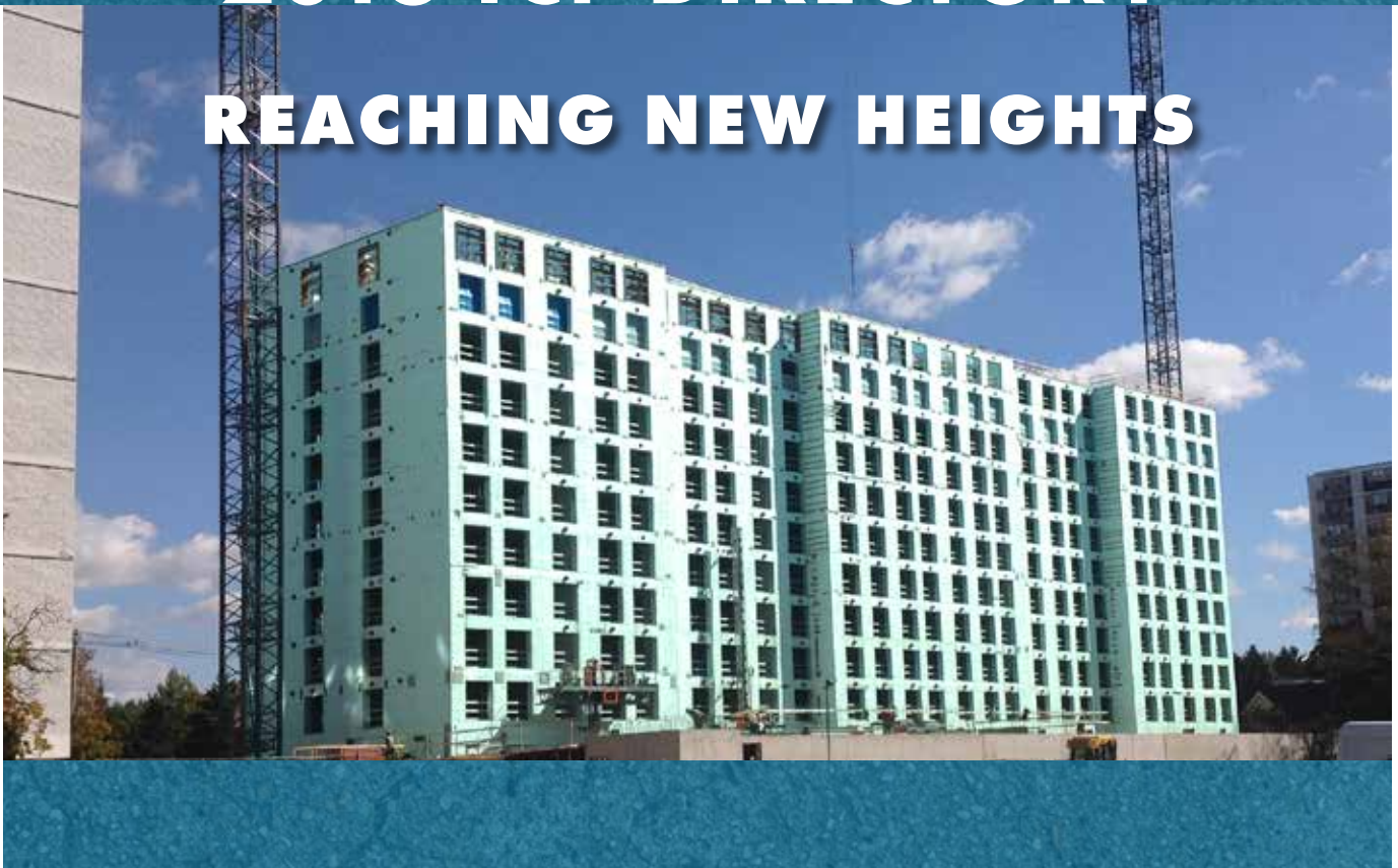
ICF construction underway at the Richmond Street Apartments student housing in Canada, encompassing 337,000 sq. ft. in 19 above-ground stories. Photo courtesy Nudura.
