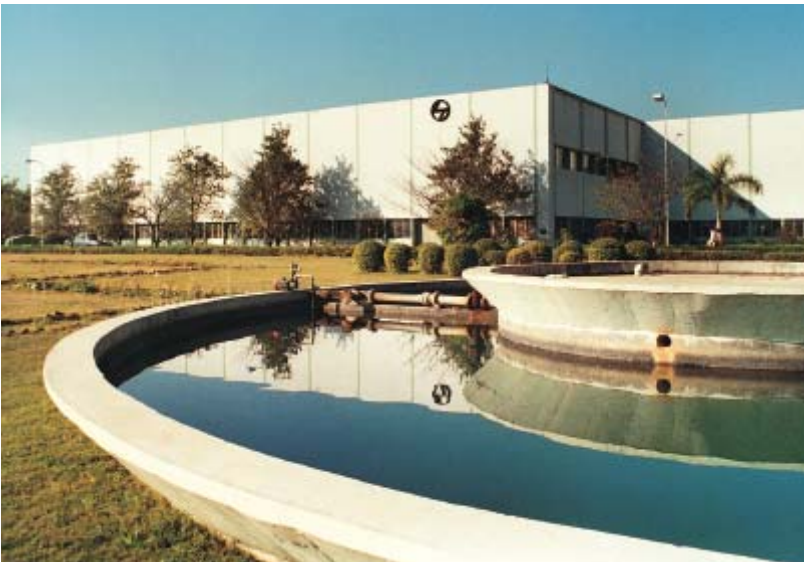
Switchgear Factory, Ahmednagar
