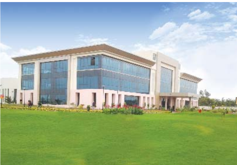
Switchgear Factory, Vadodara
