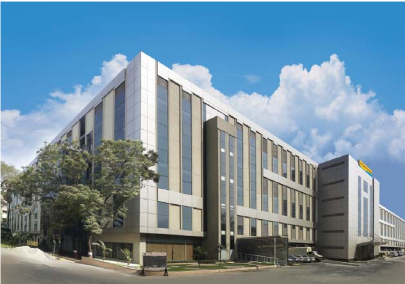
Switchgear Factory, Mumbai
