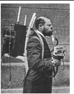
**Figure 9**. Ambulatory respirometer demonstrated by a German physiologist, Nathan Zuntz in 1906. A near term objective in the Army RT-PSM program is to provide a less intrusive version of the Zuntz metabolic monitoring capability.
