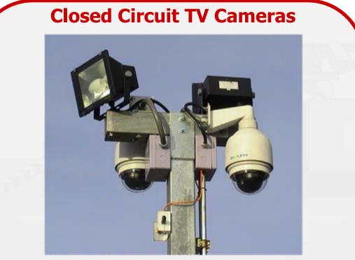
For capturing images of containers, analyze and recognize the Container ID number automatically, and also for capturing images of drivers, vehicle plate numbers for security
