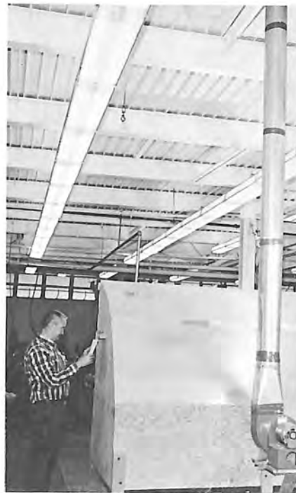
Figure 3. Vented collection hood for indoor spraying of corrosive liquids. Photo P801D-74368 NA
