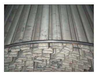
Figure 12 PJFF internal photo (Cushing and others, 2008)
