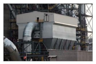
As shown in Chapter 3 there are many techniques to improve the performance of ESP. However, a FF can ensure >99% collection efficiencies of the fine particulates and >99.95% overall collection efficiency. All the information in Section 4.1 is referenced from Soud (1995) and Zhu (2003), unless otherwise referenced. Figure 10 shows a typical FF installation at a PCC plant.
