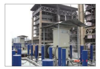
Figure 6 High frequency supply photo (Fujian LongKing, 2012)
