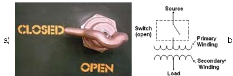
Figure 3. a) Radial Feed Switch. b) Schematic of the Radial Feed Switch.
