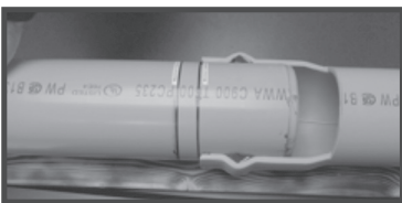
Properly Inserted Spigot
